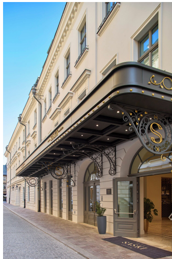
Figure 3: Photo of the Hotel Saski entrance.
